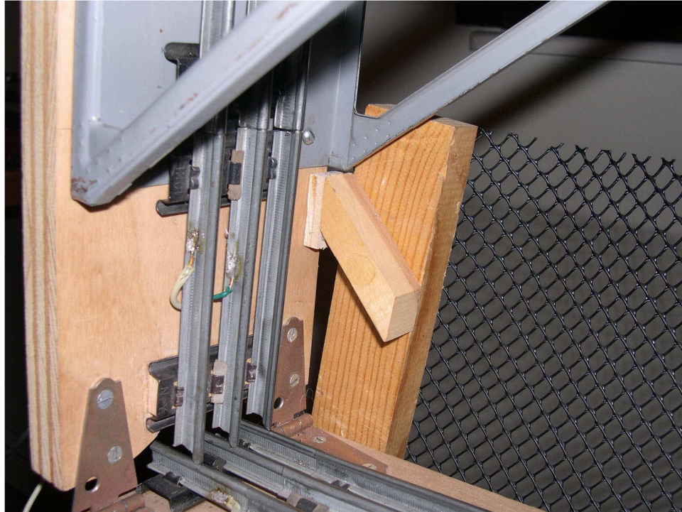
Photo #3 -- Bridge #1 - Open on stop (wooden block used for stop)
